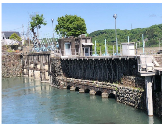
Sluice Gate No. 1 adjusts the amount of water flowing into Tamagawa Josui.
