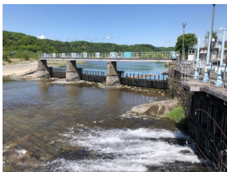
The Tama River Hamura Weir
