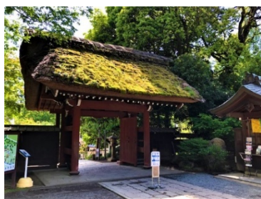
The main gate (looking back from inside)
