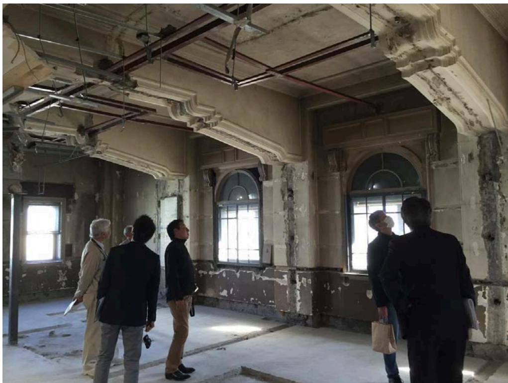
Bank under construction. Huge beams and wooden window frames emerged from the ceiling. (Photo credit: ReBITA)
