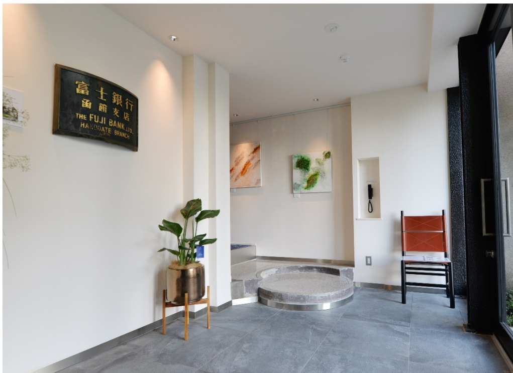
Connection point between Bank and Dock. The circular stone steps, which had been used in the time of the former hotel, were refurbished for reuse in the new facility. (Photo credit: Nikkei Architecture)
