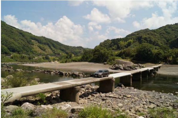
The chinkabashi is just wide enough for one vehicle to pass. The white part is a repair of part of the bridge that collapsed.
