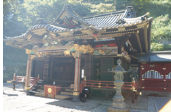
The main building of Myogi Shrine, an important cultural property of the state
